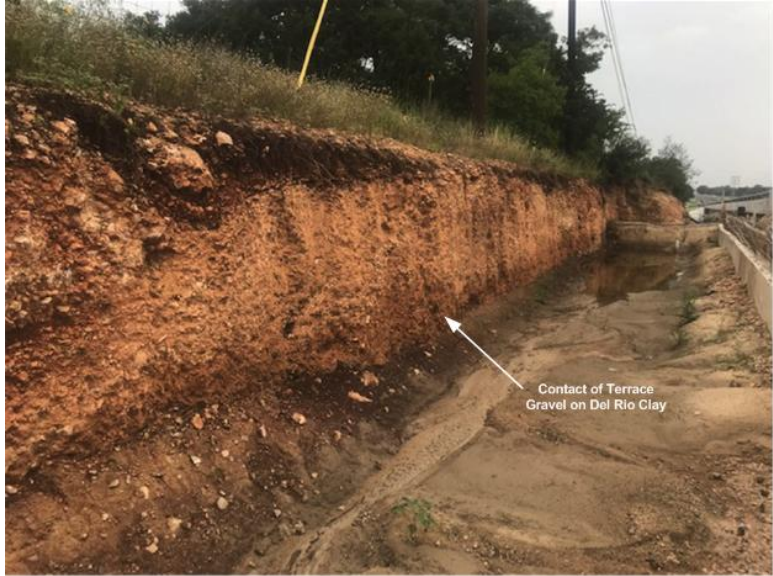
Figure 11. Roadcut Exposure of Terrace Gravel Overlying the Del Rio Clay. The FM 1626 bridge over Onion Creek can be seen on the right side of the Photo.
