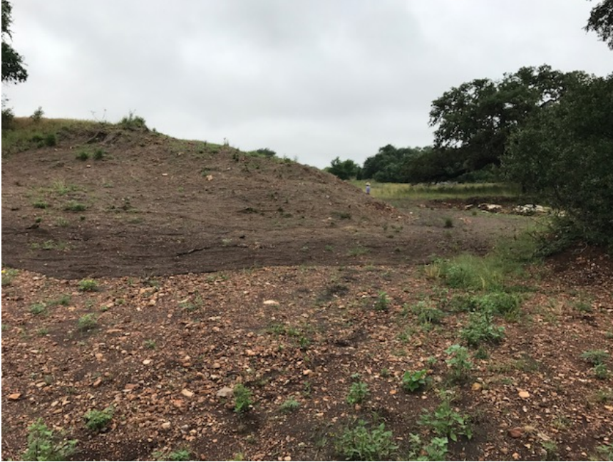
Breached Embankment, Shown on the Left, and Scoured Channel (Right) Resulting from a Flood Event.
