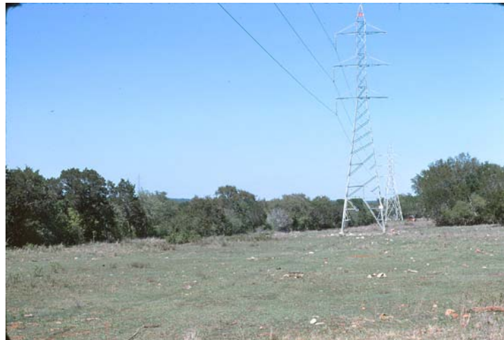
Figure 4-53. High Tension Power Line
