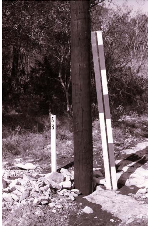
Figure 4-52. Power Pole in Limestone Substrate
