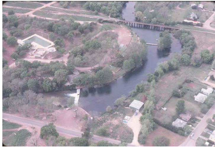
Figure 4-29. Rogers Dam and Associated Works
