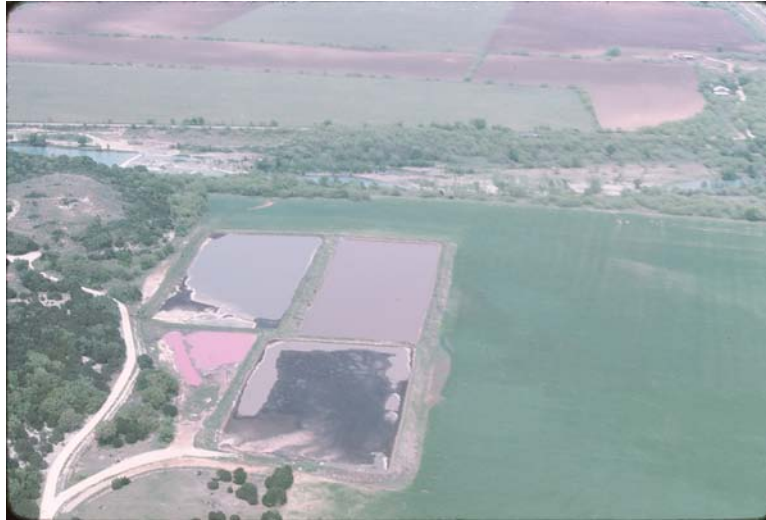
Figure 4-42. Industrial Liquid Waste Disposal Lagoons
