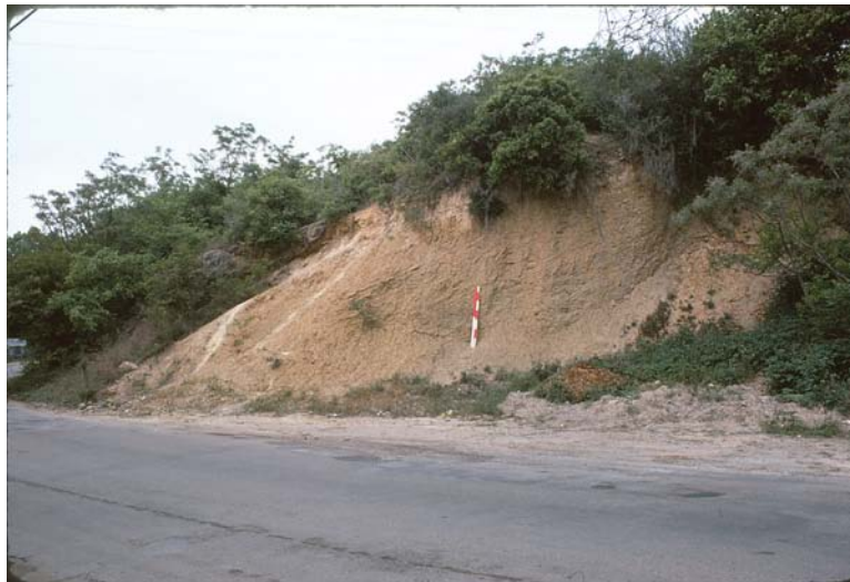
Figure 4-12. An Oversteepened but Apparently Stable Slope in the Del Rio Clay
