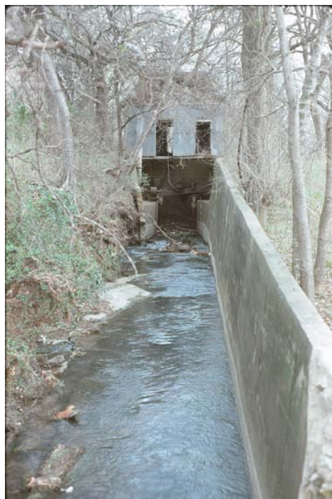
Figure 4-29. Rogers Dam and Associated Works
