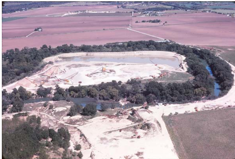
Figure 4-17. Wet-operation Sand and Gravel Pits
