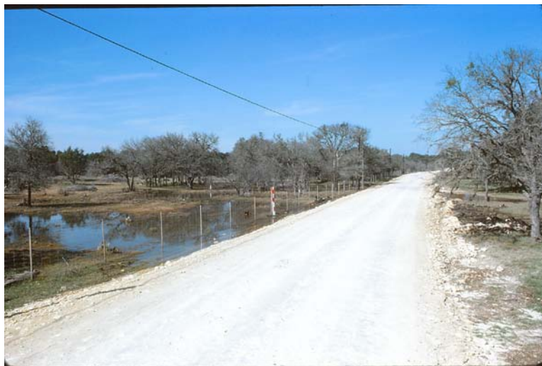
Figure 4-44. Road Constructed across Edge of Sinkhole
