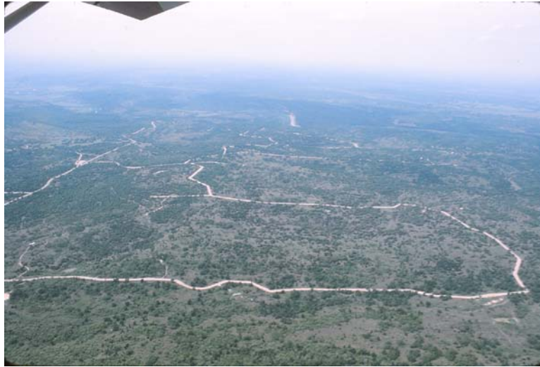
Figure 4-43. Road Network Under Construction for Outlying Housing Development
