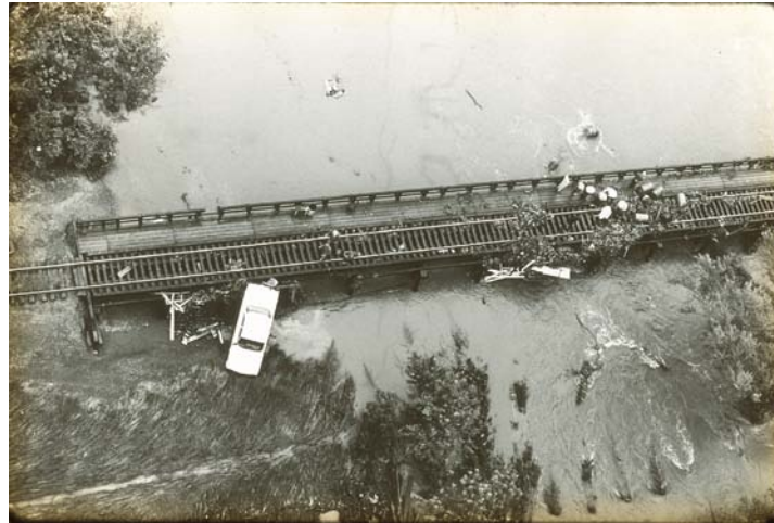
Figure 4-48. Railroad Bridge over the San Marcos River During the 1970 Flood
