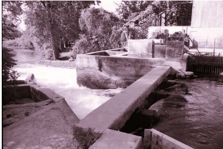
Figure 4-28. Structure Remaining from a Power Generating Plant on Spring Lake Dam
