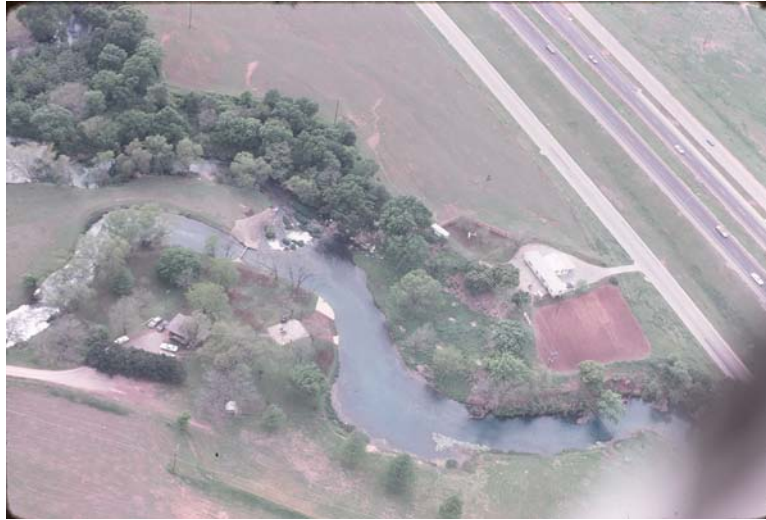
Figure 4-30. Upper Cape Dam and Associated Canal
