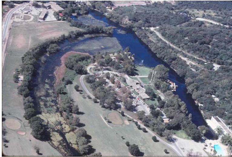
Figure 4-27. Spring Lake and Spring Lake Dam
