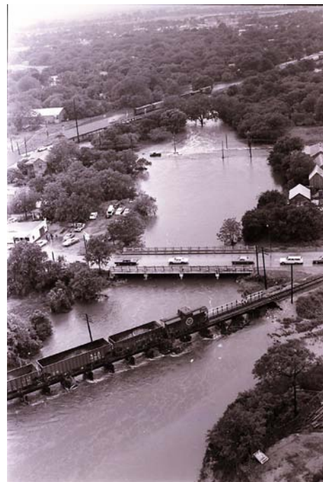
Figure 4-49. Protection of Railroad Bridges from Flood Forces by Loading Them with Freight Cars
