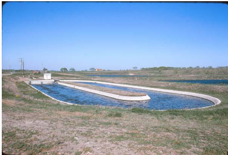
Figure 4-41. Sewage Treatment Plants in the San Marcos Area
