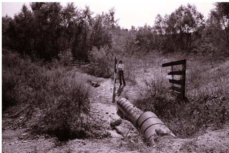
Figure 4-19. Use of an Abandoned Gravel Pit as a Silt Trap
