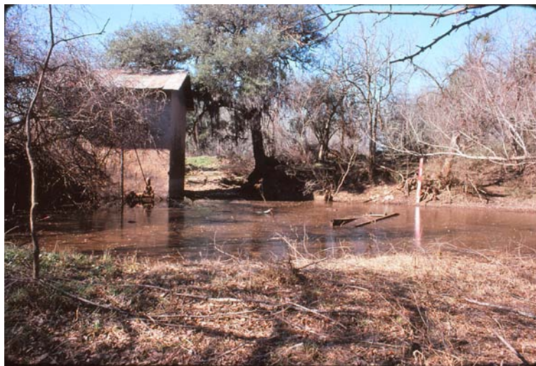
Figure 4-26. Pumphouse at Sink Springs
