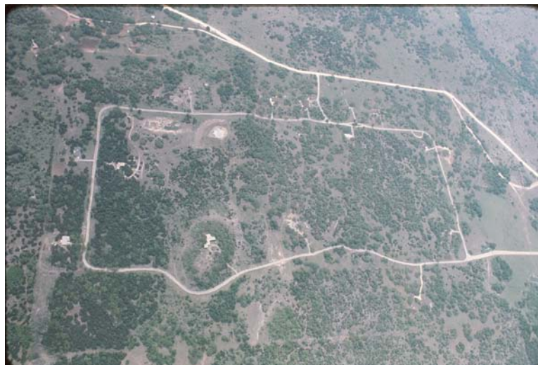
Figure 4-4. Outlying Housing Development
