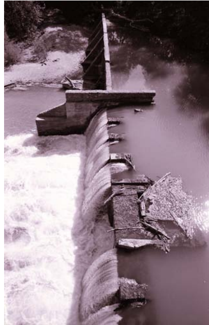
Figure 4-31. Alvord Dam and Associated Works
