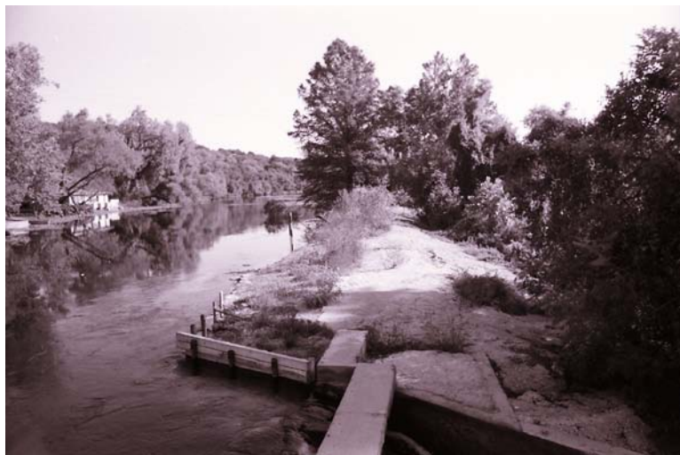
Figure 4-27. Spring Lake and Spring Lake Dam
