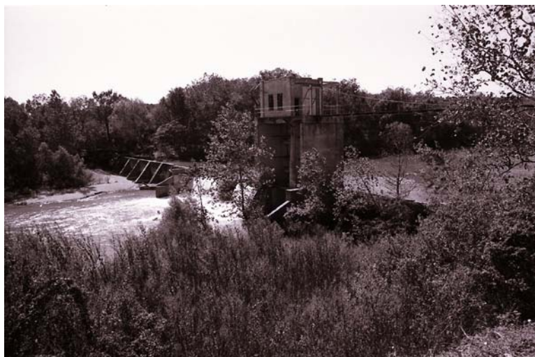
Figure 4-31. Alvord Dam and Associated Works
