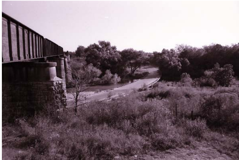
Figure 4-47. Railroad Bridge and Low-Water Highway Bridge Across the Blanco River
