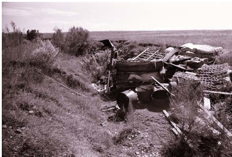
Figure 4-34. Use of an Individual Dump to Retard Erosion
